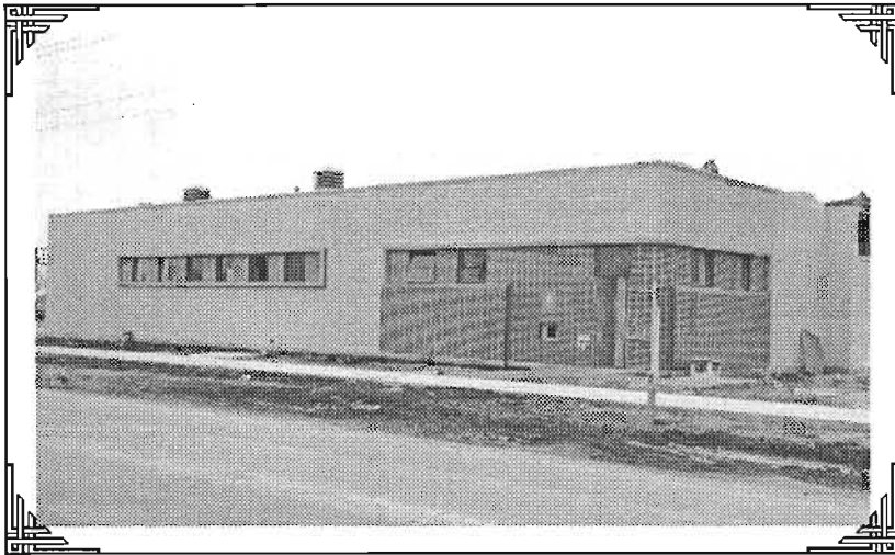
Telephone Company Dundee Road Now the garage of the telephone company
