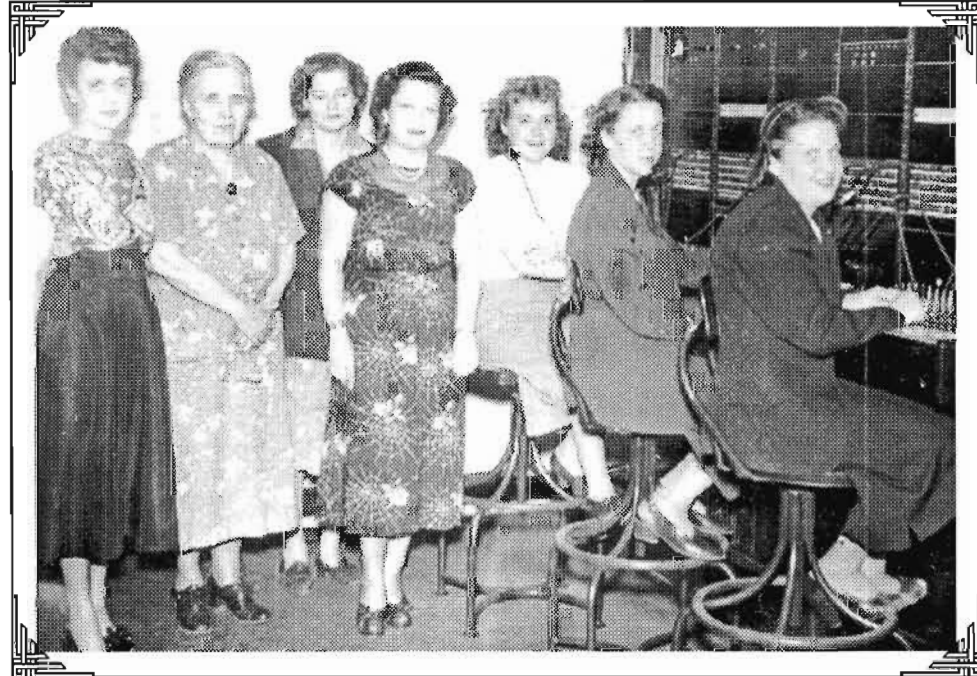
Telephone operators and switchboard
